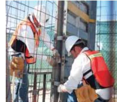
Placement of steel spacer disks
